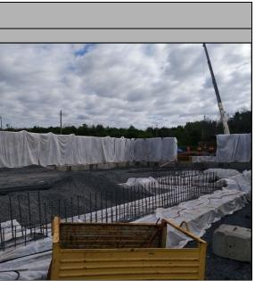
The photograph above illustrates the construction of the salt storage facility foundation and walls in progress. The concrete is covered with a membrane, which is kept wet for a minimum of seven days in order to allow the concrete to cure
