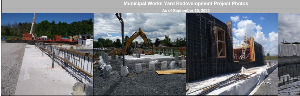
The photograph above illustrates the construction of The construction of the standby power system the proposed footings for the salt storage facility. The footings around the perimeter of the building are 4.7m in width and 0.65m in height and are reinforced with rebar throughout. The exposed rebar (as seen above) will tie into the future salt storage facility walls.
