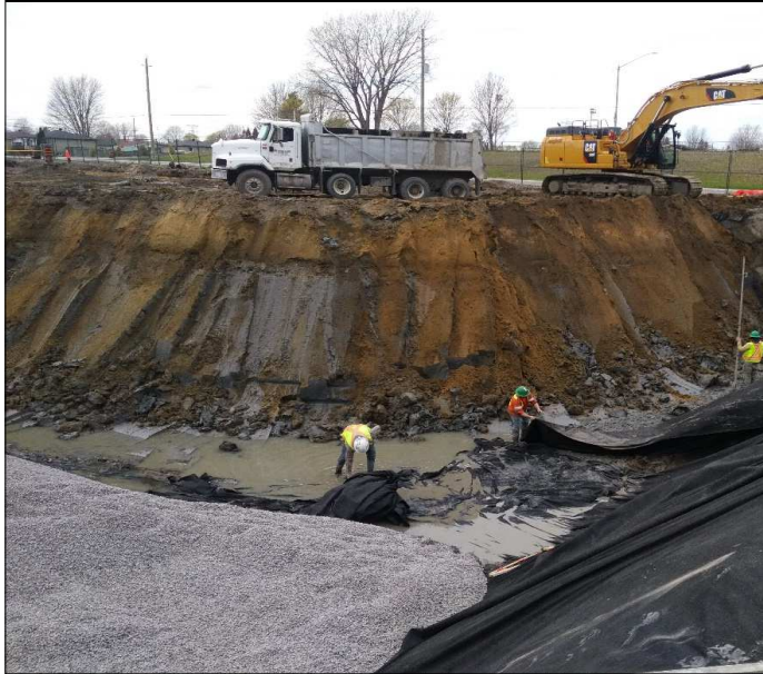
The construction of the proposed salt storage facility included a 5.5m deep excavation in order to remove soil that was not suitable for construction. Following the completion of a geotechnical review in 2018, it was estimated that up to one (1) metre of settlement was likely to occur if the proposed building was constructed on the existing soil in lieu of excavating to suitable subgrade as shown above.
