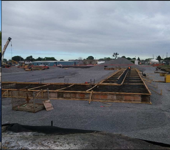
In June, 2020 the Contractor began forming the proposed footings for the salt storage facility. The footings around the perimeter of the building are 4.7m in width and 0.65m in height and are reinforced with rebar throughout.
