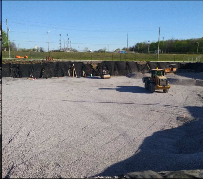
The clear stone engineered fill foundation was placed and compacted in 0.6m lifts, as indicated in the photo above. The building footprint area for the proposed salt storage facility is approximately 60m long by 30m wide.
