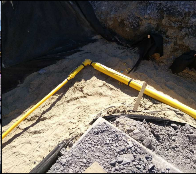
As part of the first phase of redevelopment within the MW Yard, a new 100mm polyethylene gas main was installed. The new gas main will service all existing/future buildings within the MW Yard. The photo above depicts where the 100mm main branches off with a 32mm gas main in order to service the existing MW Garage.
