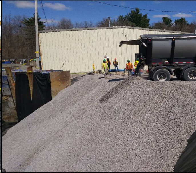
The excavated area for the salt storage facility was backfilled with approximately 29,000 tonnes of clear crushed stone. The clear stone is considered a light weight engineered fill, which will act as a suitable base for constructing the salt storage facility on.
