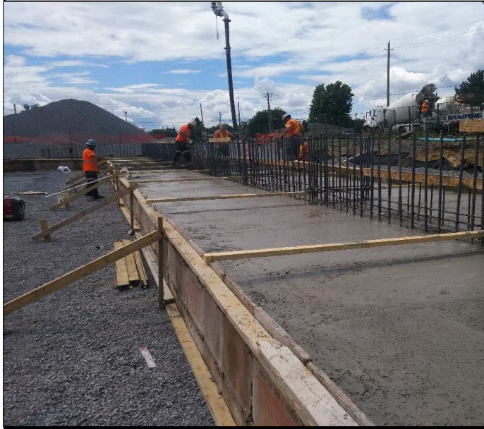
The photograph above was taken during a concrete pour for the foundation footings. As specified in the previous photograph description, the footings are 0.65m in height and 4.7m wide. The rebar visible in the centre of the footing is where the future foundation walls will tie into the footing.
