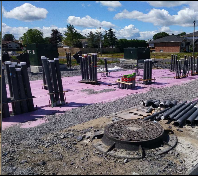
As part of the preparatory work required in order to install the precast buildings within the utility compound, the Contractor placed rigid insulation in the area surrounding the buildings and stubbed up all the conduit that lead to each of the three (3) pre-cast buildings. In July, 2020 a crane will be brought on site to lower the buildings in place in order to ensure that the conduit are not disturbed.
