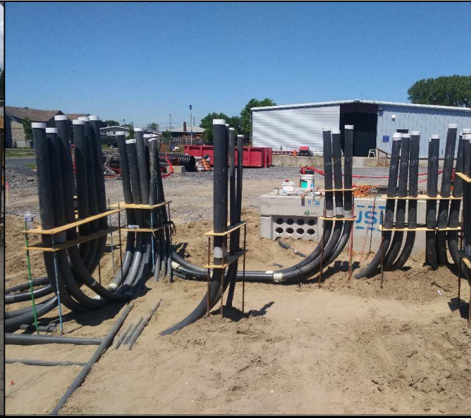
The photograph above illustrates the conduit that will be located in the precast buildings within the utility compound. The conduit will be directed from the utility buildings to the various (proposed) buildings within the MW Yard. The conduit installed are part of the long term plan for servicing and will be used for both electrical connections and communications.
