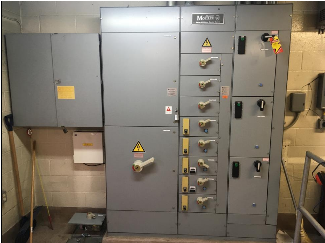
Figure 3: Motor Control Centre Layout
