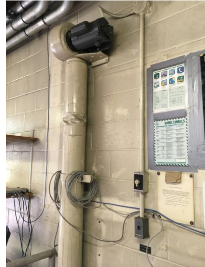
Figure 45: Wet Well Air Blower
