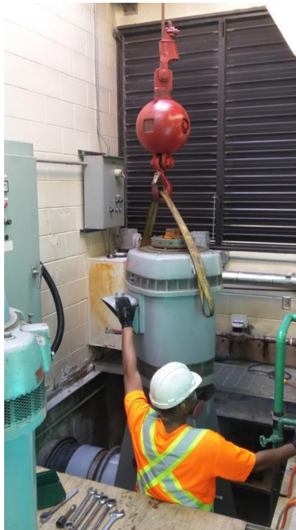
Figure 22: Pump 3 - Motor Re-install
