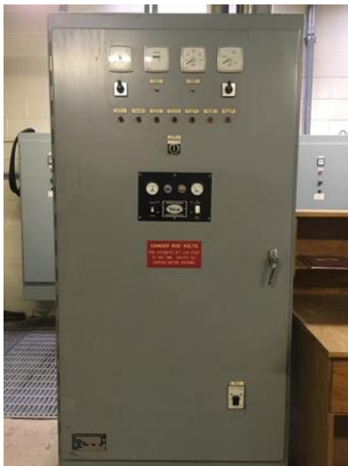
Figure 35: Automatic Transfer Switch
