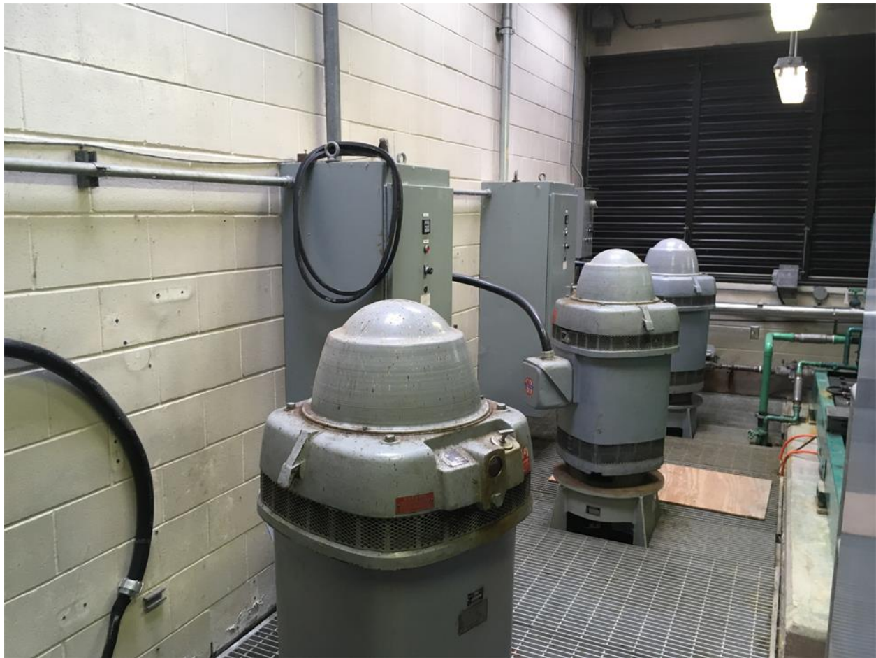
Figure 8: Main Pumps and Motors
