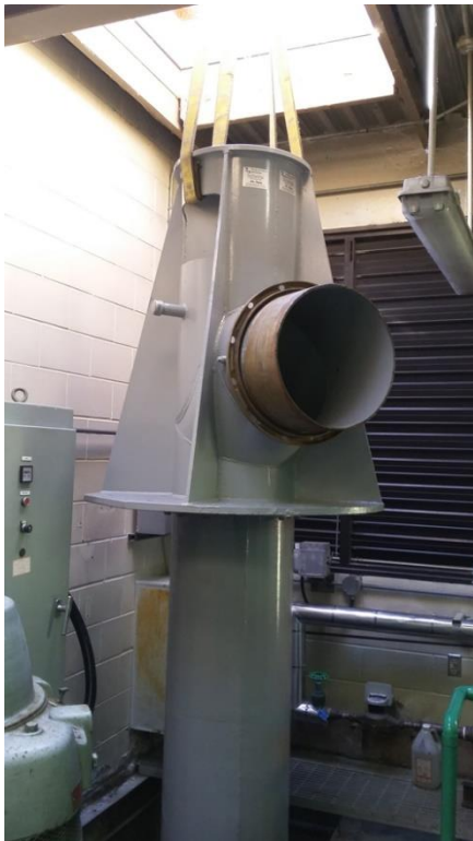
Figure 21: Pump 3 - Casing Re-install
