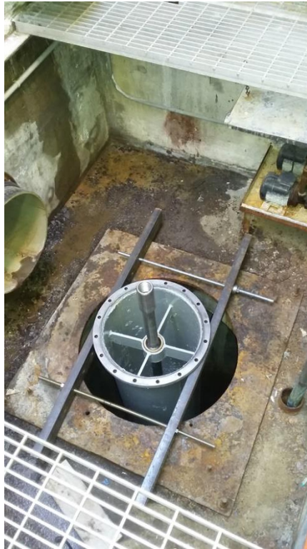
Figure 22: Pump 3 - Motor Re-install
