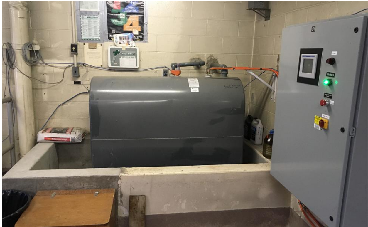
Figure 38: Diesel Fuel Tank
