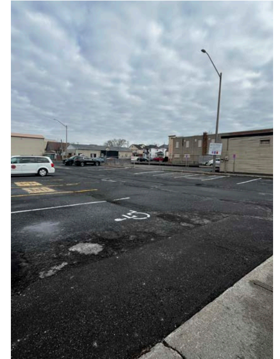
Existing parking area
