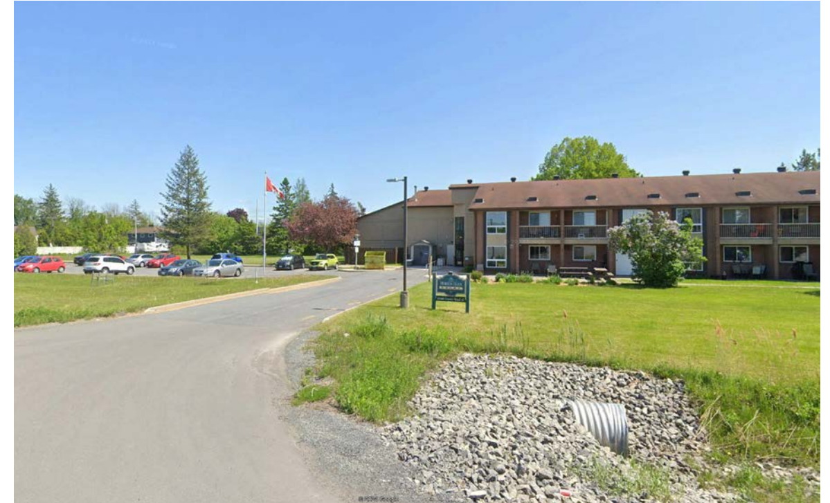
View looking south along County Rd 2
