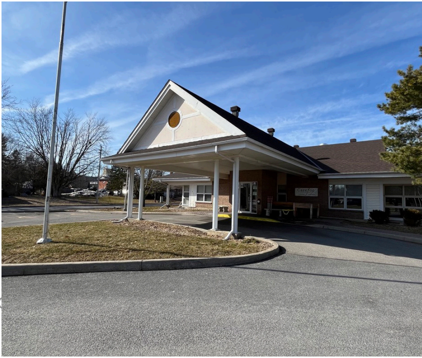
View looking north towards Seniors Support Centre
