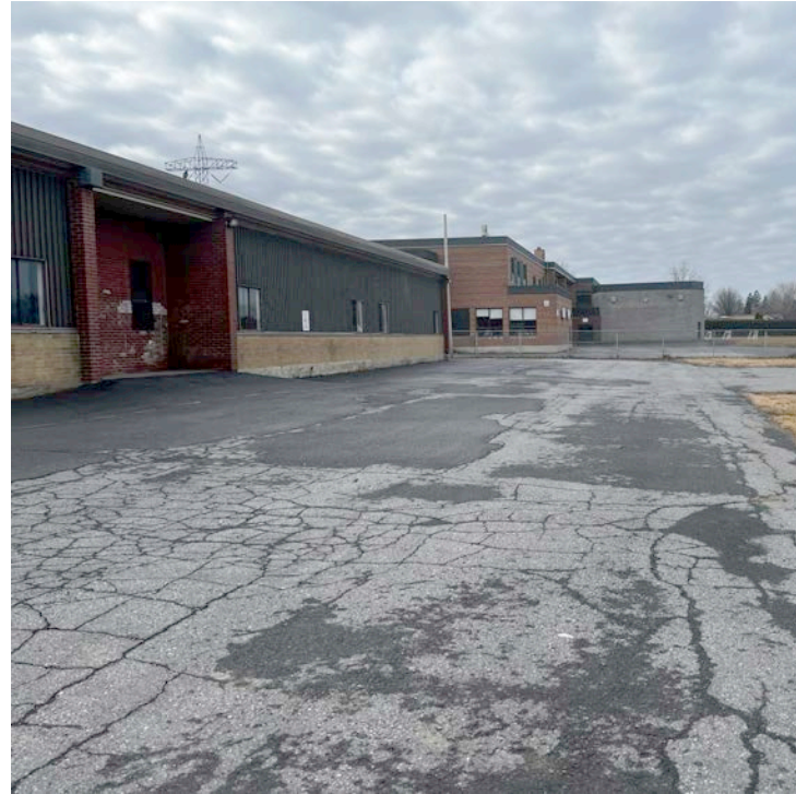
View looking southeast along existing parking lot
