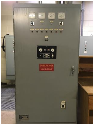
Figure 35: Automatic Transfer Switch
