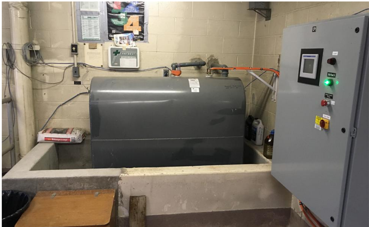
Figure 38: Diesel Fuel Tank
