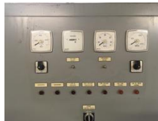
Figure 37: Transfer Switch Gauges
