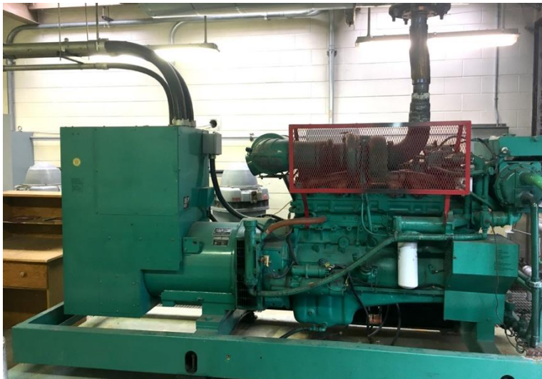
Figure 33: Cummins Diesel Engine
