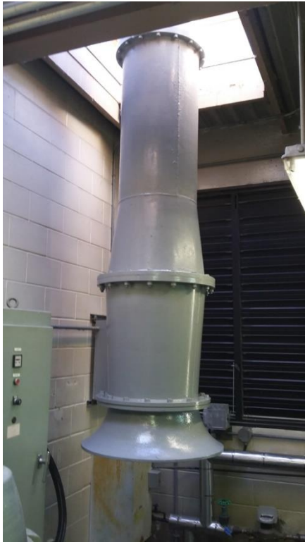
Figure 21: Pump 3 - Casing Re-install
