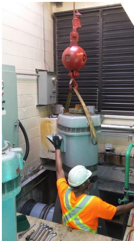
Figure 22: Pump 3 - Motor Re-install
