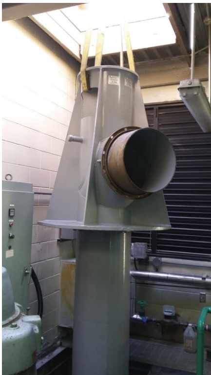
Figure 21: Pump 3 - Casing Re-install
