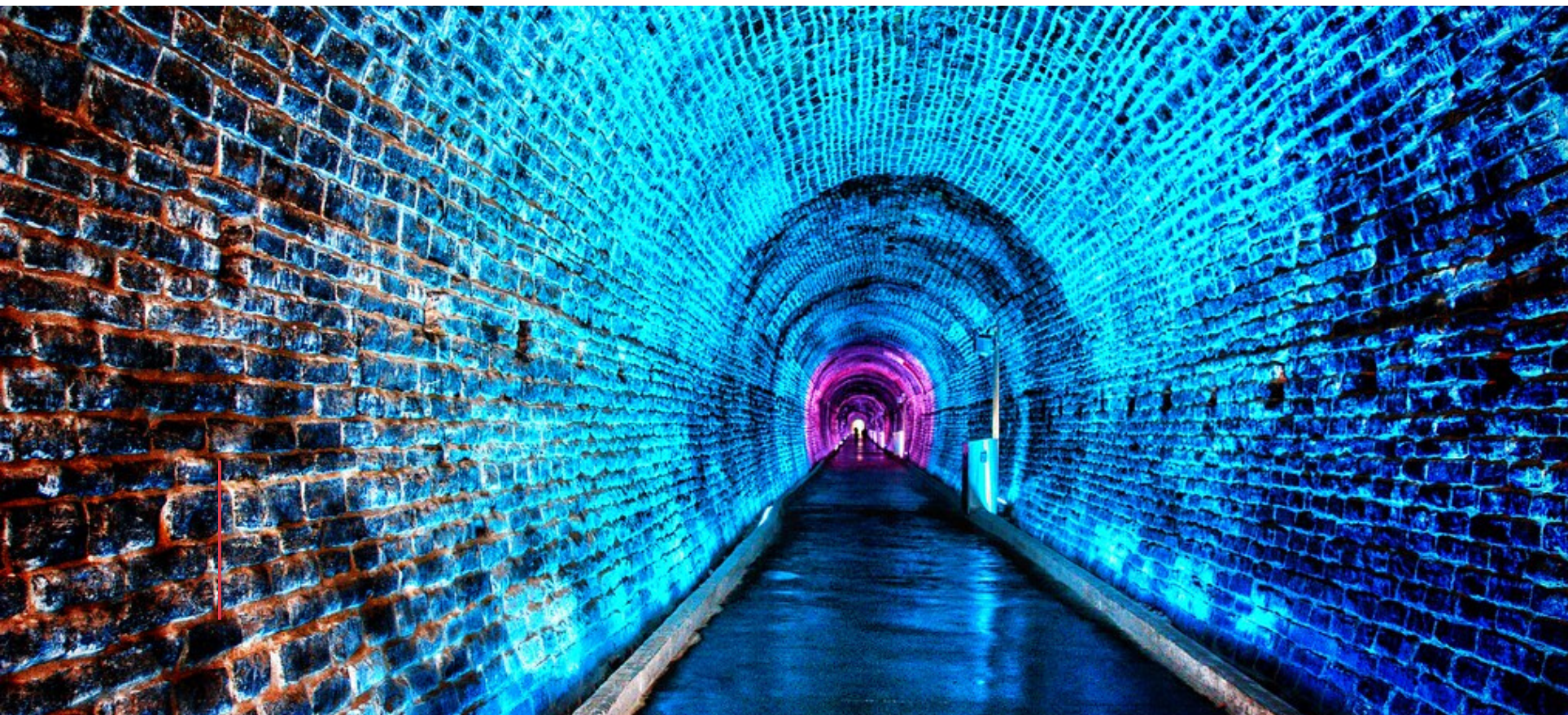
Brockville Light Tunnel
