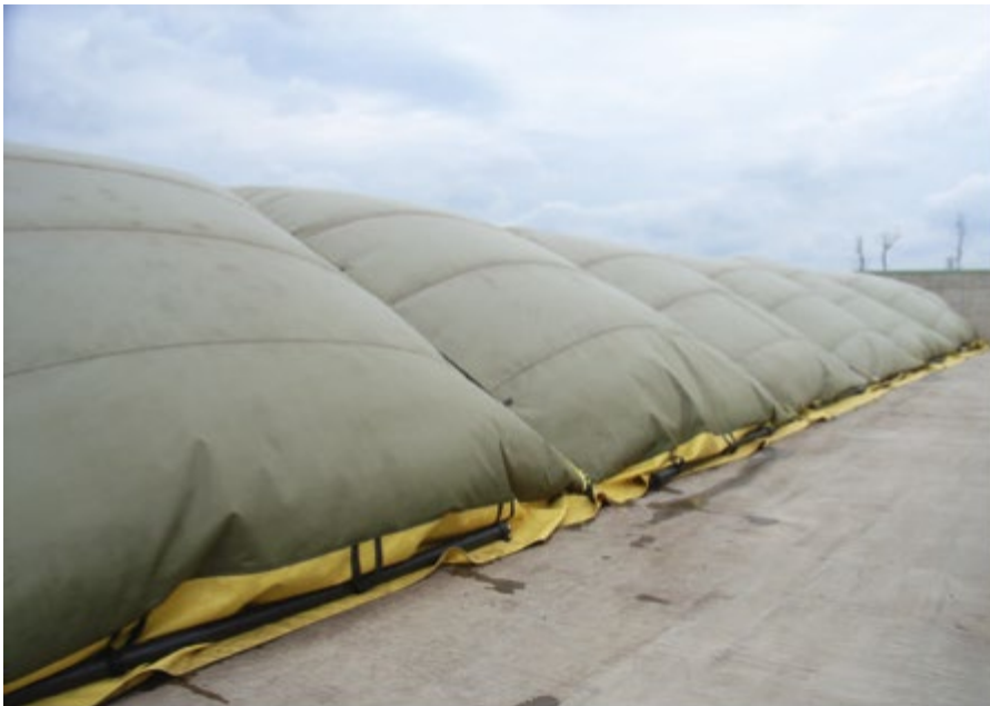
Figure 4.10 Example Covered Composting System for approximately 20,000 tonnes per year located in Moncton, NB (Courtesy of W.L. Gore & Associates)
