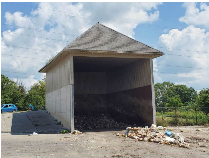
Figure 4.9 Example Organic Food Waste Receiving Building (Cambridge Waste Management Centre, Cambridge, ON)
